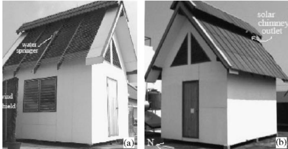
Fig. 2-6 Módulos experimentales con chimenea solar y sistema de aspersores. Fuente: Chungloo, S. y Limmeechokchai, B. (2006) Application of passive cooling systems in the hot and humid climate: The case study of a solar chimney and wetted roof in Thailand. Building and Environment No. 47 pp. 3343.
