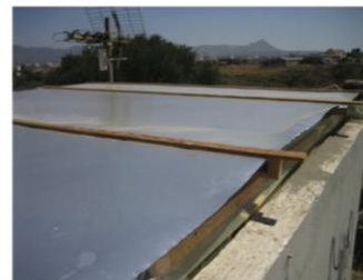
Fig. 7. The tested device: ventilated pond covered with aluminium.
