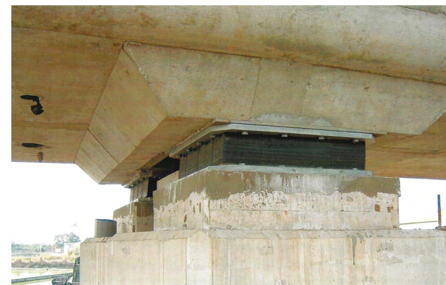
SEISM INSULATOR. MAGEBA COMPANY PHOTO
