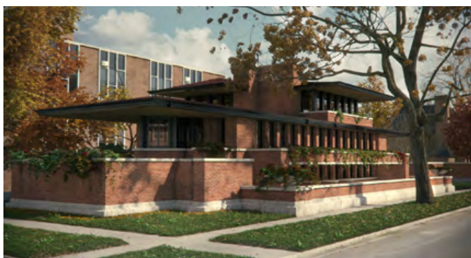
Figura 39. Frank Lloyd Wright. Casa Robie. Fachada principal sur (orig06.deviantart.net/5e8a/f/2012/301/c/2/robie_house_by_7y8i-d5j8ils.jpg).
