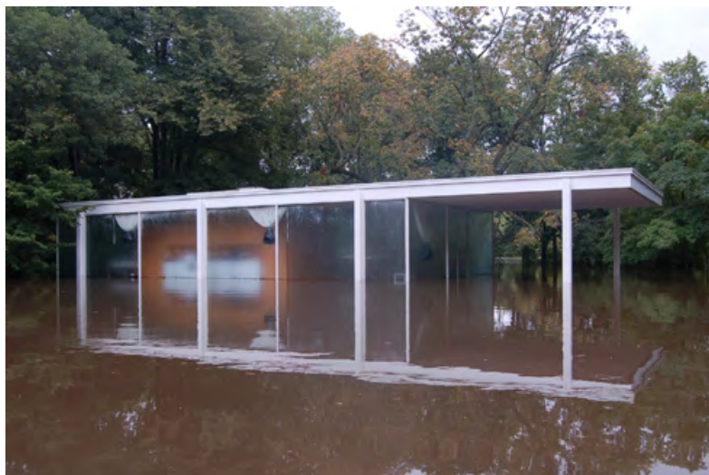
Figura 38. Mies van der Rohe. Inundación de la casa Fransworth ( www.archdaily.com/770612/a-virtual-look-into-mies-van-der-rohes-farnsworth-house/55afa85ae58e6c07000145-a-virtual-look-into-mies-van-der-rohes-farnsworth-house-image ).
