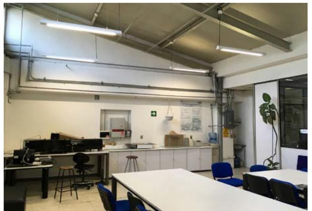
Image of the light installation in the Bioclimatic Architecture laboratory. Example of surrounding illumination of high uniformity.
