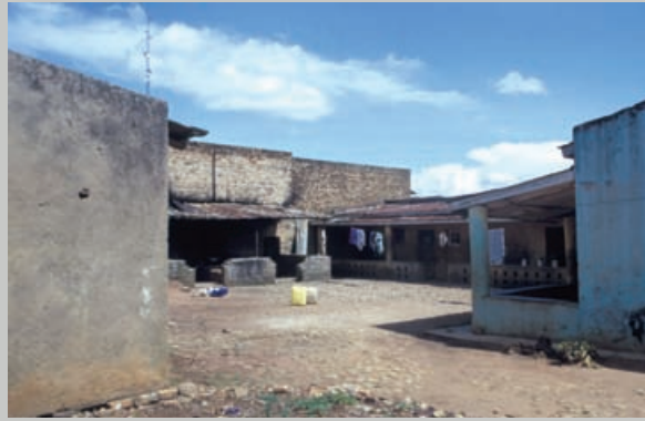
Figure 46. Second courtyard of the double courtyard typology.
