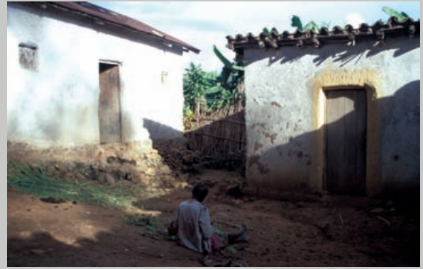
Figure 43. Courtyard of one house.
