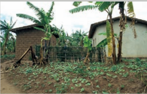
Figure 39. Courtyard house, Nyanza.
