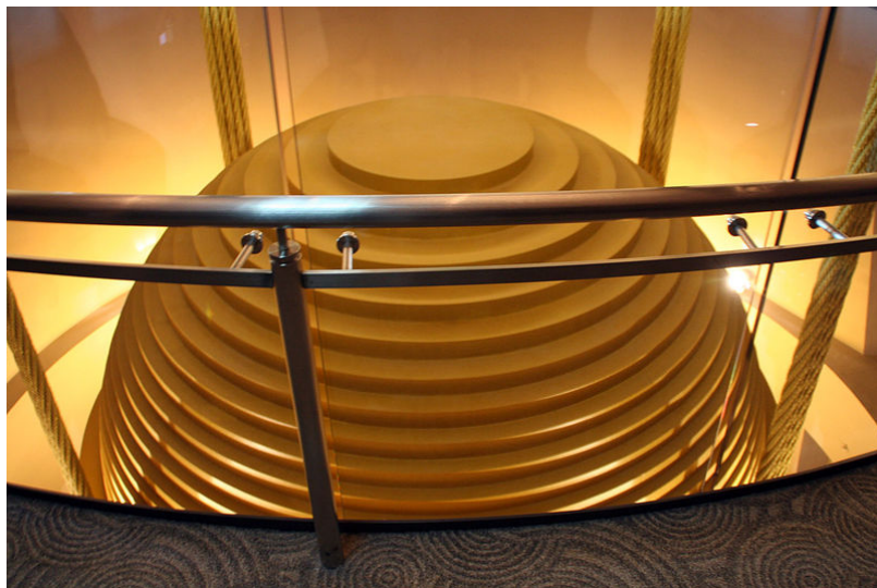
Figure 1.2 TMD instalada en Taipei 101 ( http://wikipedia.org )
