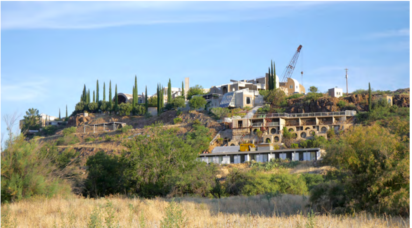
Figura 43. Paolo Soleri. Arcosanti. Vista general (By Carwil, Own work, CC BY-SA 4.0, https://commons.wikimedia.org/w/index.php?curid=60360895 ).
