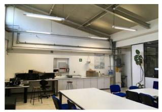
Image of the light installation in the Bioclimatic Architecture laboratory. Example of surrounding illumination of high uniformity.
